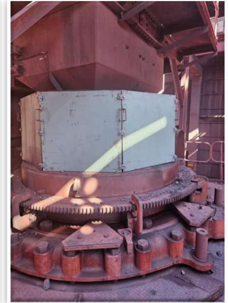
After installation of noise acoustic material
