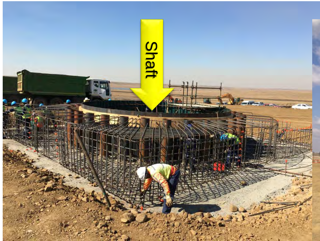
Upcast Shaft Construction
