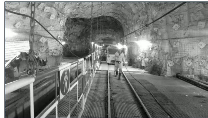
Pedestrian with cap lamp – Tracking lost, warning zone
