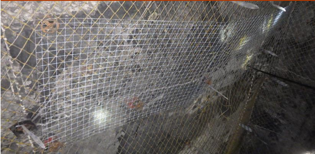
Systemic roof welded mesh support pattern using double nuts/Q-links
