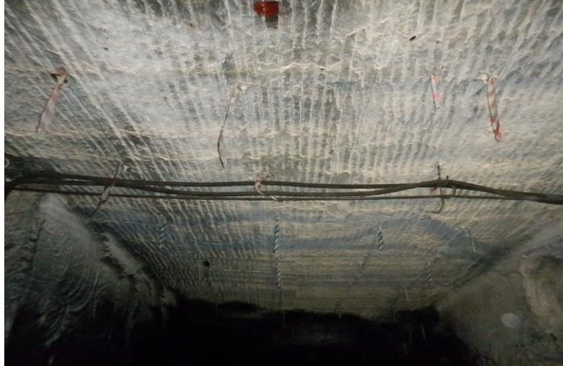
4 x 1.8m x 20mm full column resin bolts
