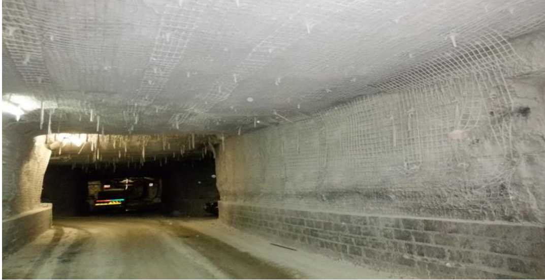
Systemic roof and sidewall welded mesh support pattern
