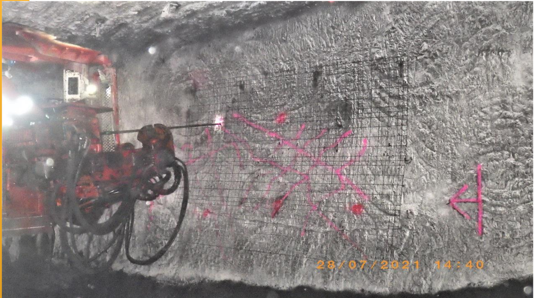
Image 8: Mesh placed, ready for bolting.
