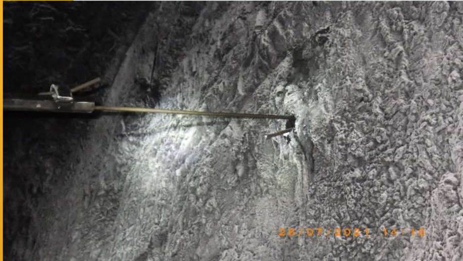
Images 4 and 5: Inserting the Z-Hook.
