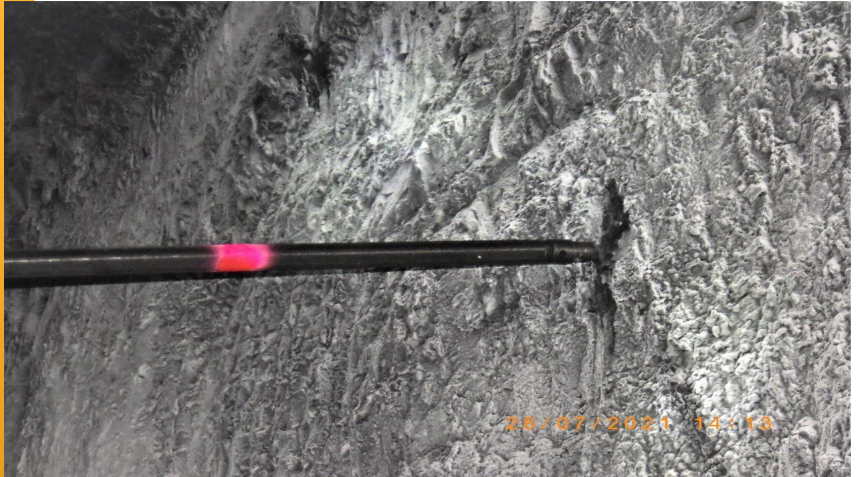
Image 2: Marking of correct drill depth and drilling Z-Hook holes.
