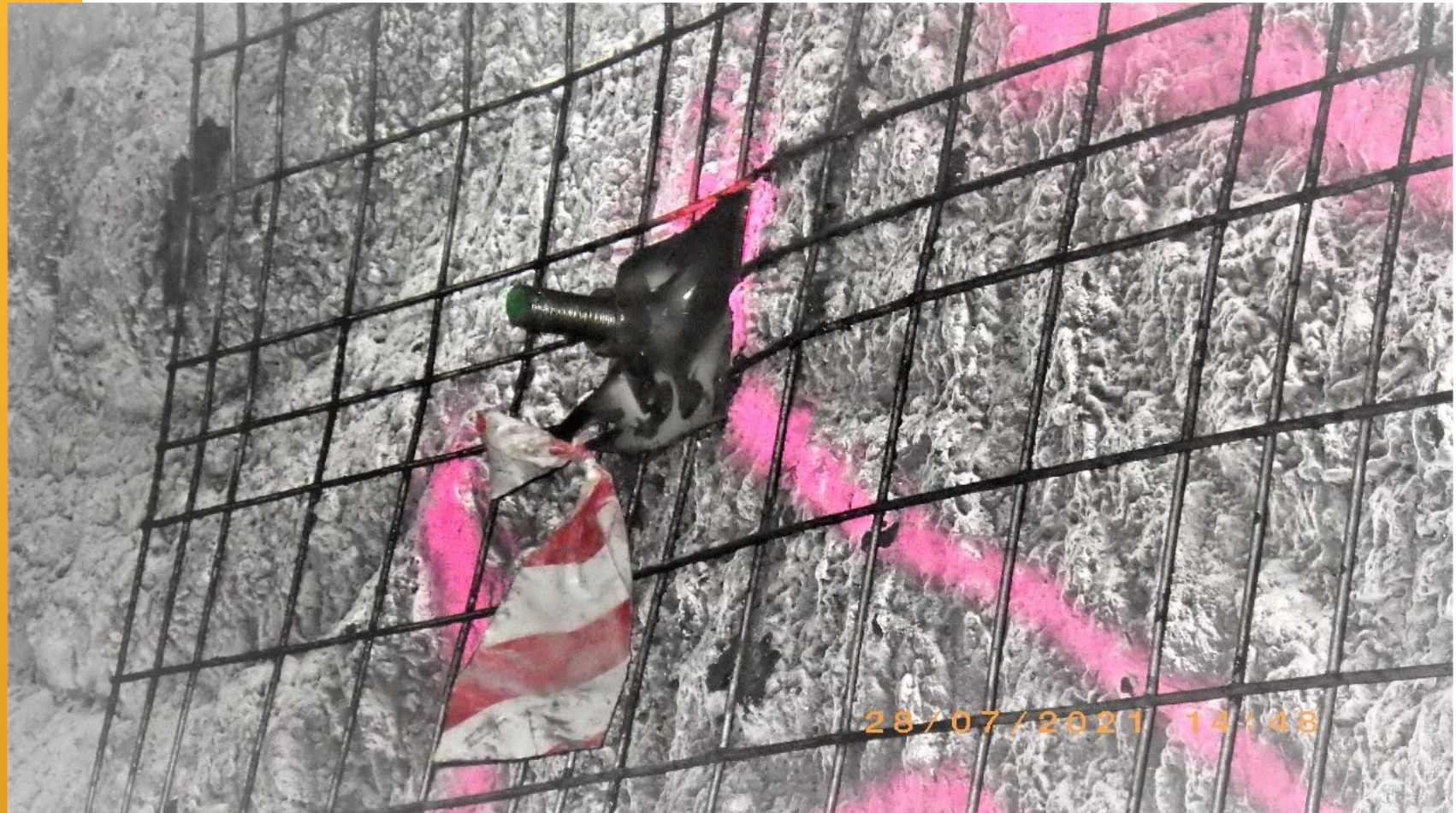
Image 9: Mesh bolted, area made safe.
