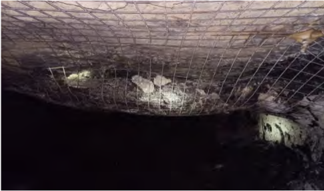
Figure 1: Photographs indicating loaded (left) and overloaded (right) mesh conditions
