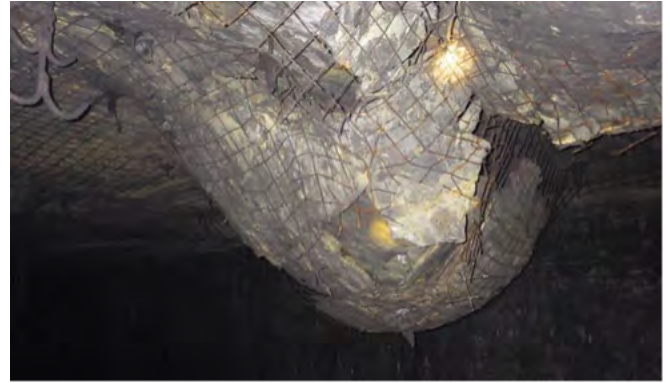
Figure 1: Photographs indicating loaded (left) and overloaded (right) mesh conditions
